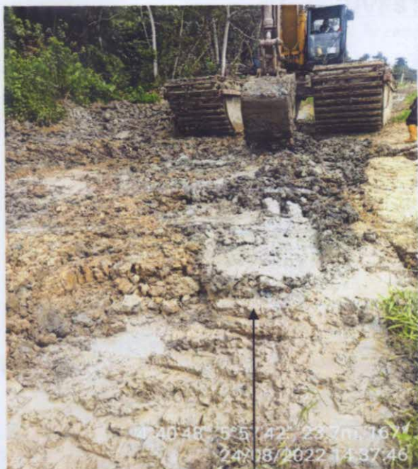
SPILL POINT BEFORE EXCAVATION
